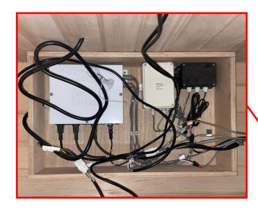
Place the electric box on the floor of the sauna and position where the bench will enclose it.
